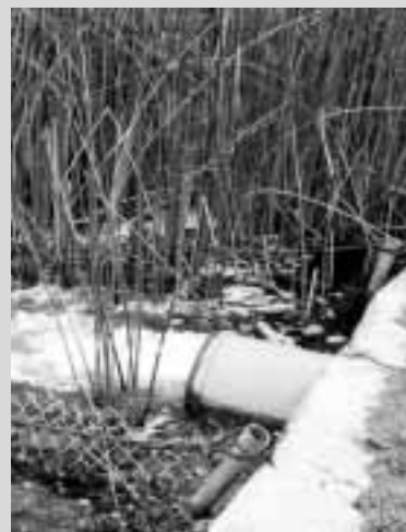
City of Orlando Streets, Drainage and Stormwater Utility
