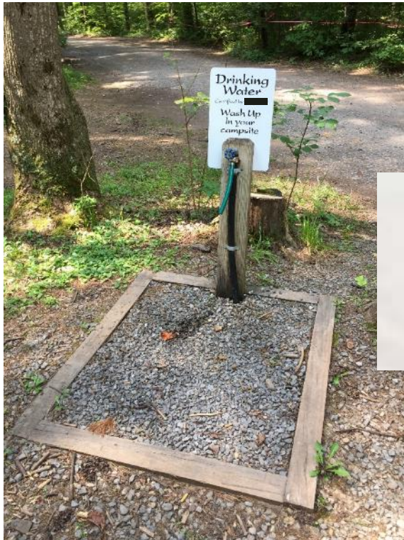
New drinking water well
