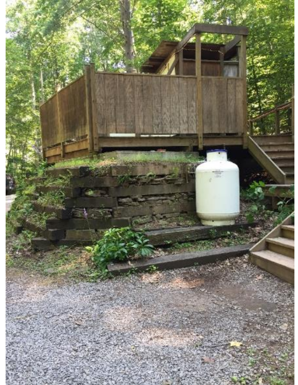
Toilet and showers connected to septic
