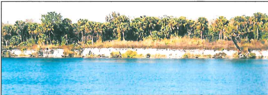
Figure 16. Side cast spoil along waterway at Rialto.
